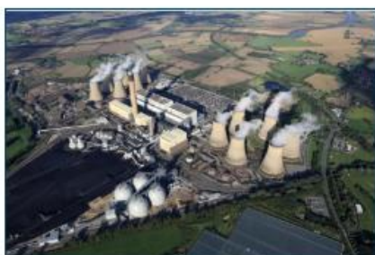
Drax Power Station
