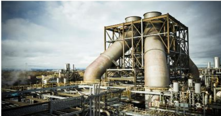
The Teesside gas-fired power station. Photograph: Alamy
