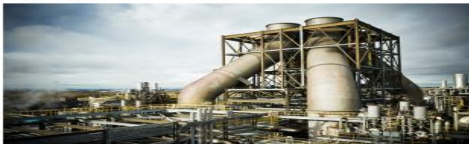
▲ The Teesside gas-fired power station. Photograph: Alanay
